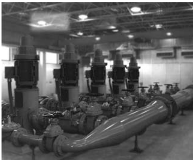
Figure C6.17 Multiple pump installation
